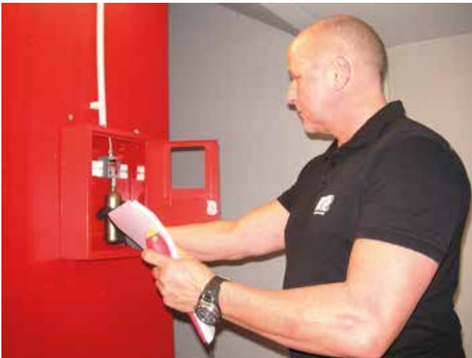
Sachkundige Wartung einer RWA-Anlage Expert maintenance of an SHE system
